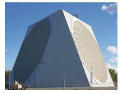
PAVE Phased Array Warning System (PAWE) radar in Alaska Intercontinental ballistic missile warning, space surveillance and sattelite tracking
